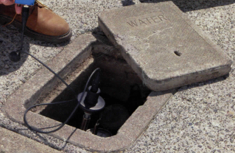
Leak Surveying with the LD-7 at a Meter Box
